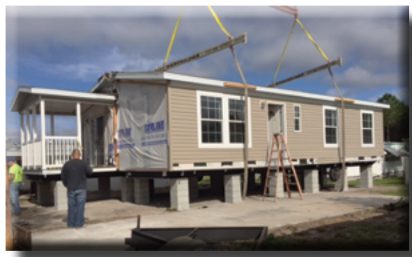
8th Street house almost put together. Lookin' good!
